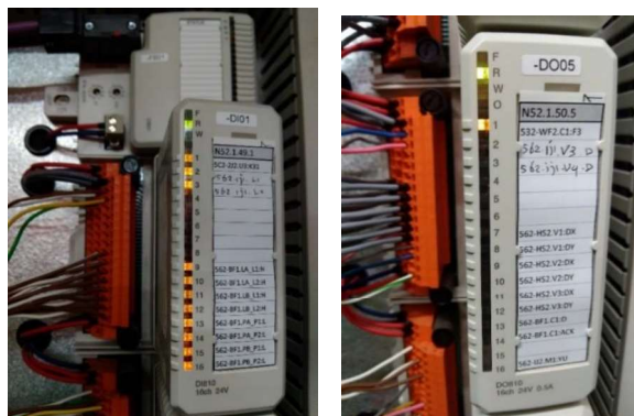
Gambar. 8 Koneksi I/O panel control valve 562-IJ1
