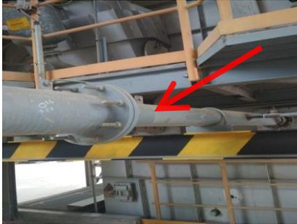
Gambar.3a Saluran Pipa Calsiner Burner
